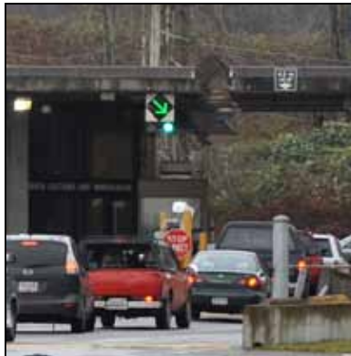
The Aldergrove Port-of-Entry
