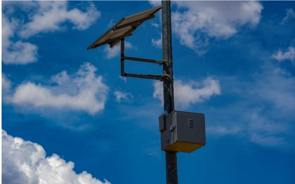
Figure 10. Bluetooth Reader Technology for BWT Measurement
