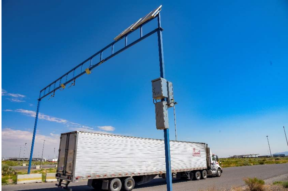
Figure 9. RFID Technology for BWT Measurement
