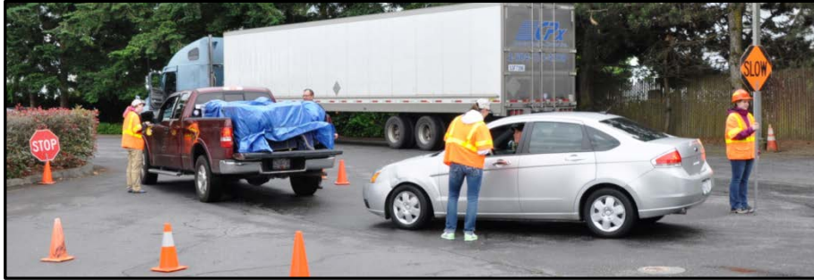
Surveying at Lynden, WA.
