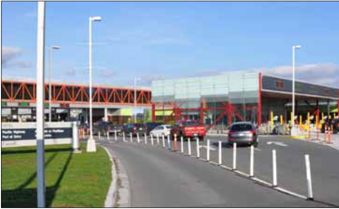
Northbound the number of inspection lanes for passenger vehicles increased to eleven in 2012.
