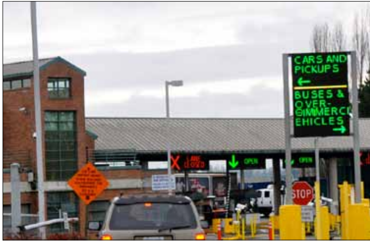
LED signage at the U.S. Lynden crossing allows for more dynamic lane management
