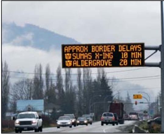
Southbound ATIS system on BC Highway 11
