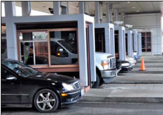
Northbound inspection booths at Pacific Highway Port-of-Entry
