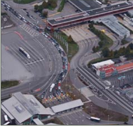
Aerial view of the U.S. and Canadian ports-of-entry at Pacific Highway
