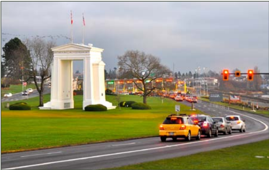
The anti-idling traffic control system at Peace Arch Port-of-Entry
