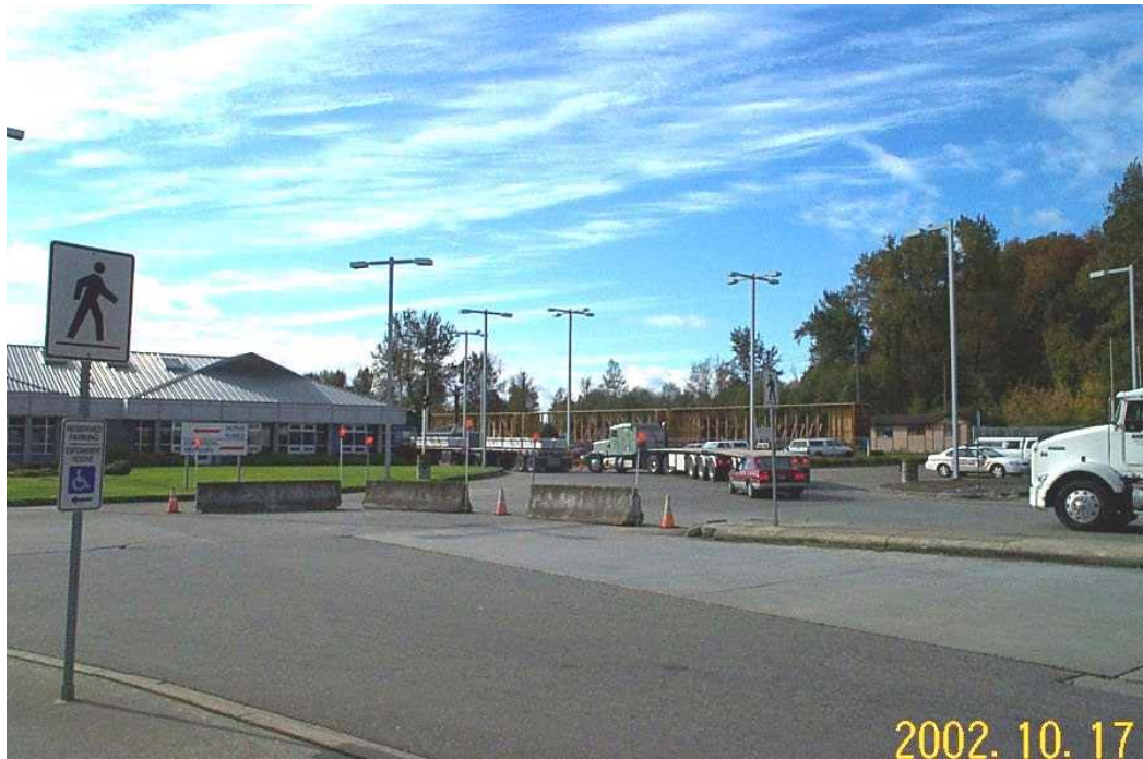
Photo 4a – Concrete roadside barrier at U.S. Customs following September 11.
