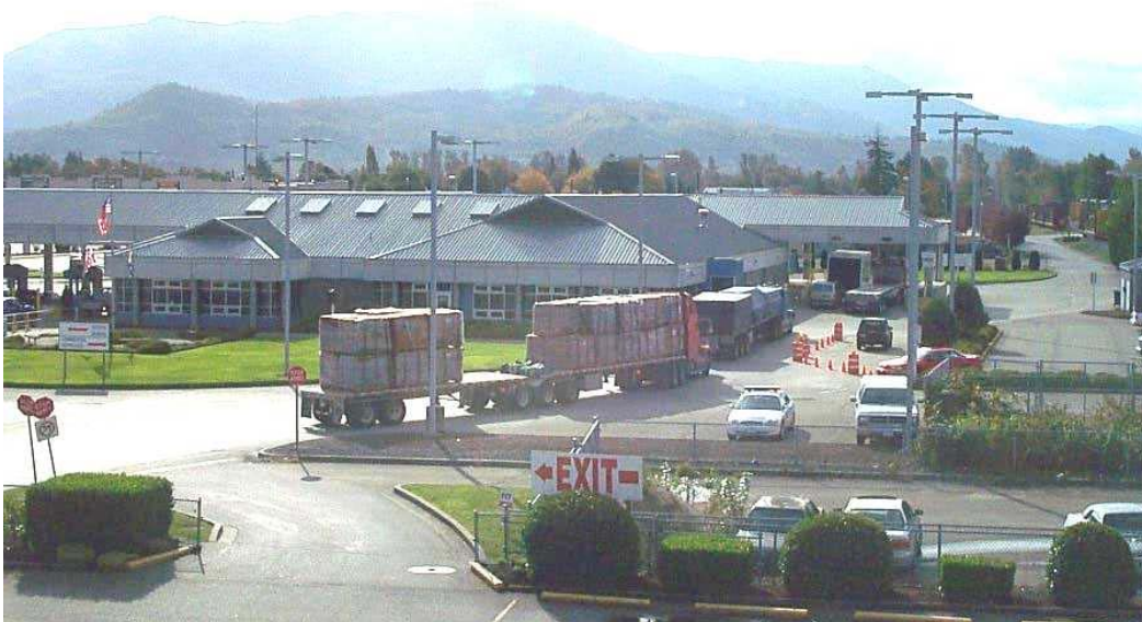
Photo 1b – Huntingdon/Sumas border crossing. Southward view of commercial vehicle inspection booth.
