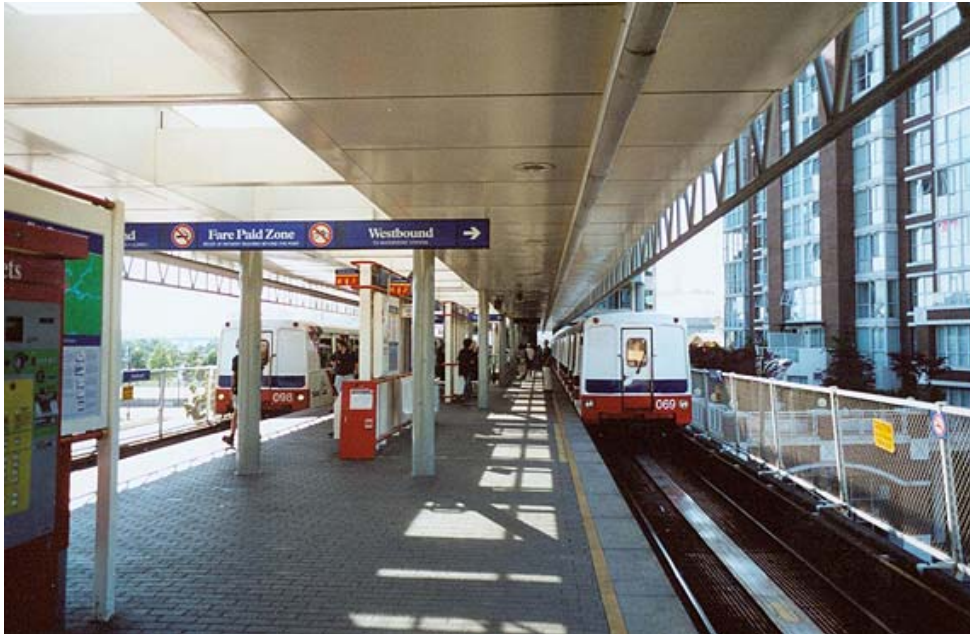
Figure 6-1 Scott Road SkyTrain Station
